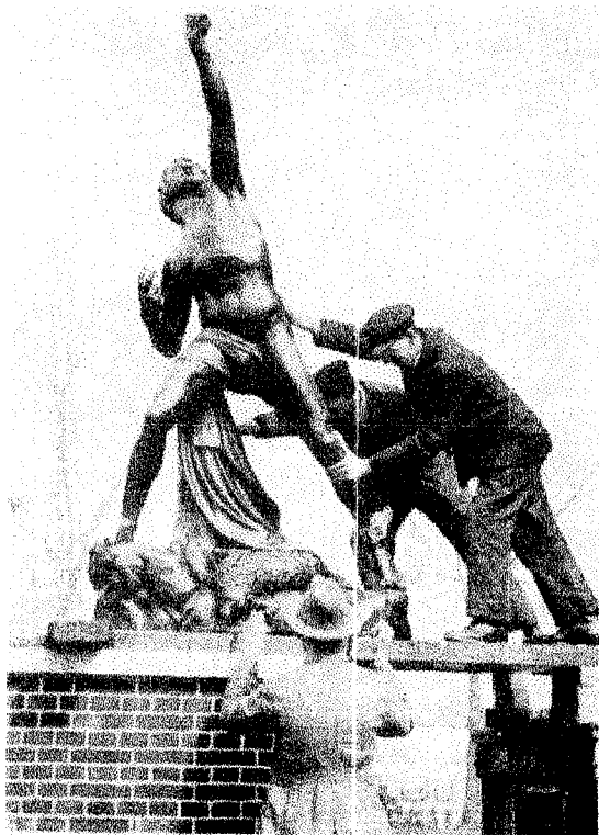
The Eagle Slayer being erected in Bethnal Green Museum Gardens in April 1927
