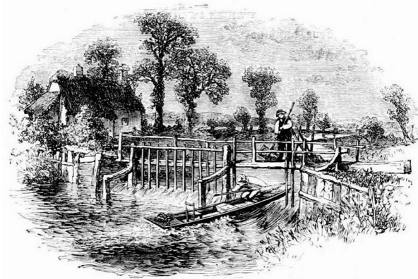
Hart’s weir (now the site of Northmoor Lock on the Thames near Oxford) – a ‘paddle and‘rymer’ weir with the ‘paddle’ raised for a boat to pass upstream through the flash lock
