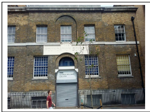
Whitechapel building in 2019
