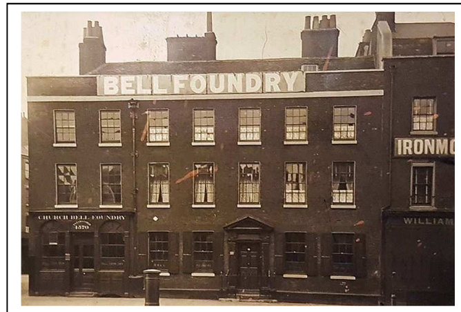
Whitechapel Bell Foundry frontage in 1906
