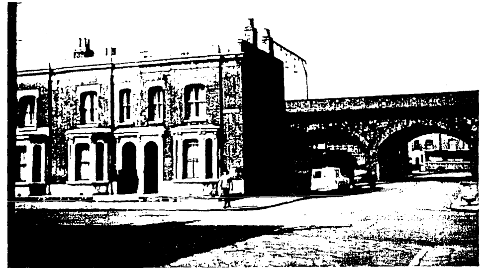
A view of the 1960s looking N.W. (from point ① on the map), towards 165 Turners Road, Bromley, and the Robeson Street arch of the (early 1850s) Blackwall Extension Railway.
